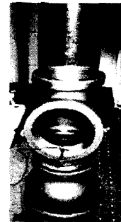
Figure 1: The lower portion of the duct, with "T" section and grid of burner visible
